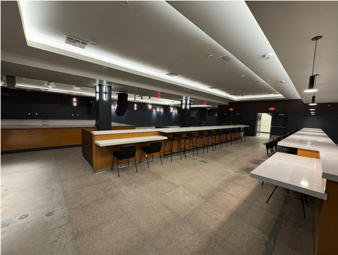
Photograph 9 Woolworth Building, Basement Level. Event venue and bar, view southeast.
