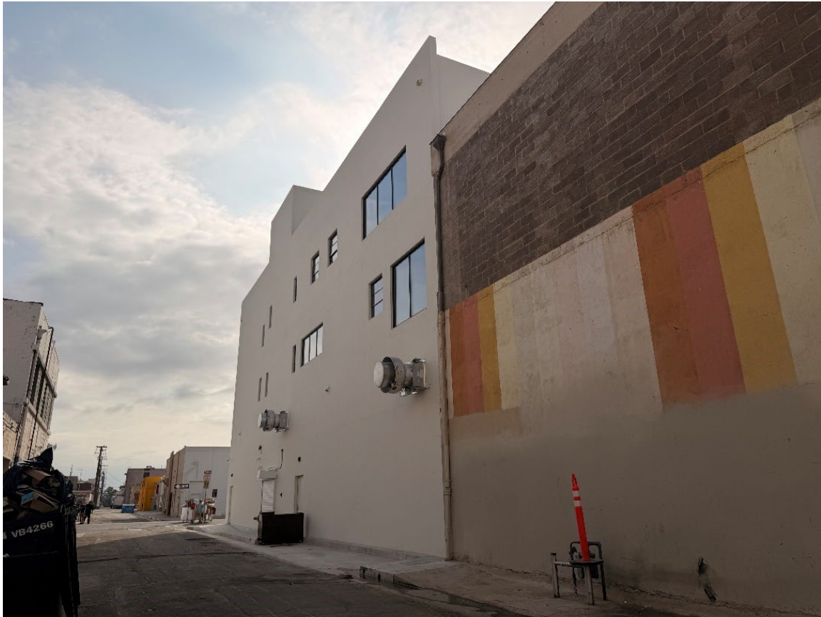
Photograph 4 Woolworth Building, oblique view of rear (north) façade, looking southeast.
