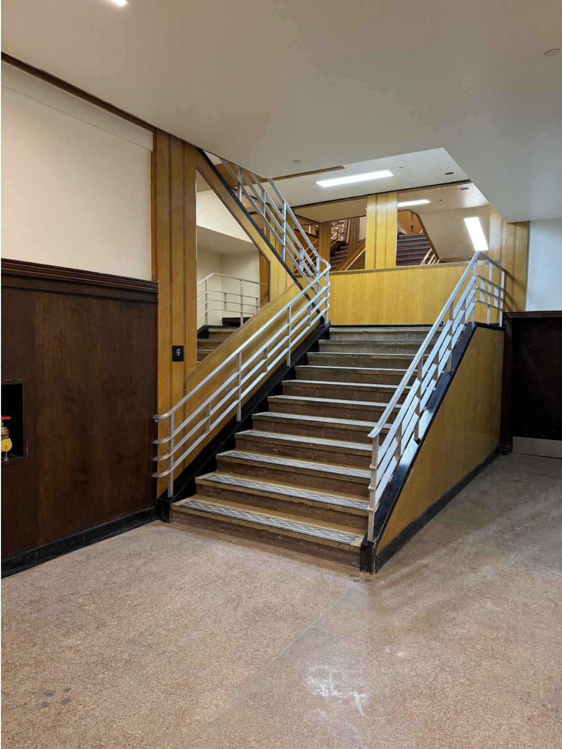
Photograph 8 Woolworth Building, Basement Level. Detail of Stair 2, looking east.
