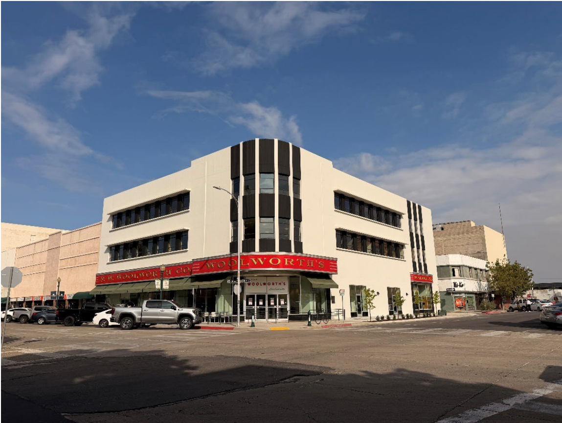
Photograph 1 View of the Woolworth Building showing curved corner and both south and east primary façades. Looking northwest.
