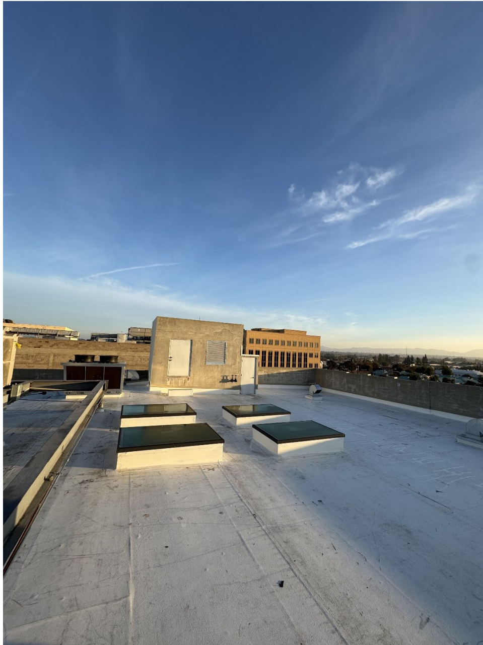
Photograph 21 Woolworth Building, Roof. New skylights and exit stair penthouse, view northeast.
