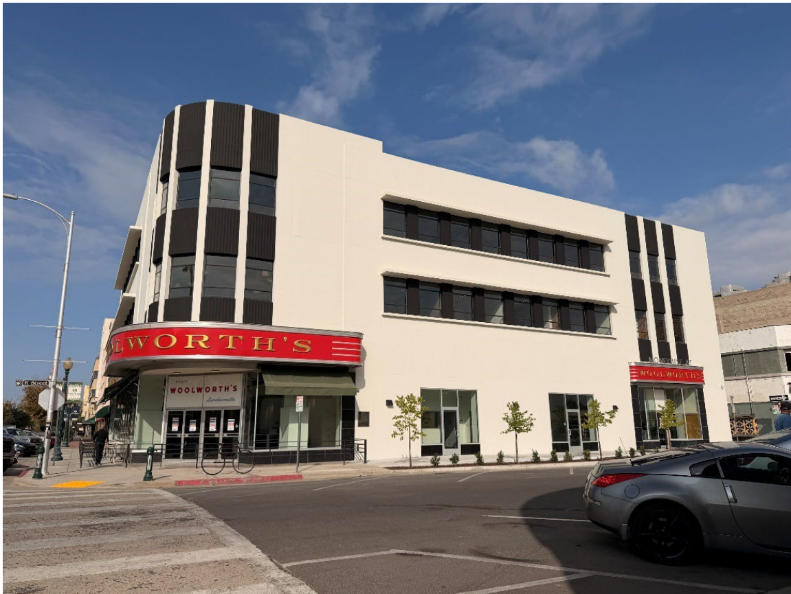
Photograph 2 Woolworth Building, primary (east) façade, looking northwest.
